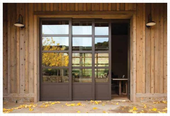
Liftslide Doors, like this, are our highest-performing big doors. When the door is closed it lowers onto seals that help provide air and water protection.
